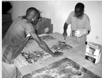
Making acoustical absorber panels for the new recording studio.
