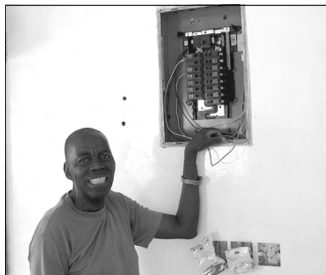
Baba Steven, installing the circuit breaker box for the Community Center.
