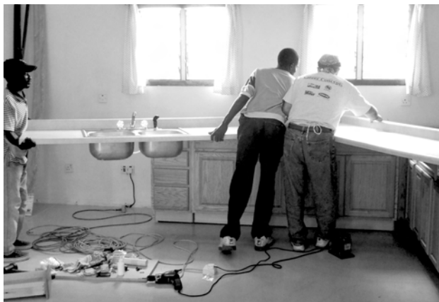
Vance installs the new kitchen in the Calvin guest house.
