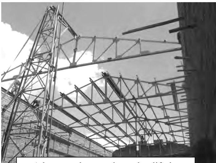
A homemade crane is used to lift the trusses into place.
