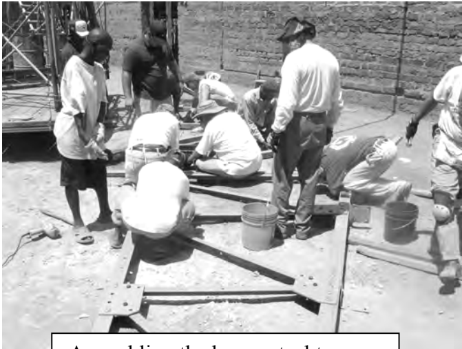
Assembling the heavy steel trusses.
