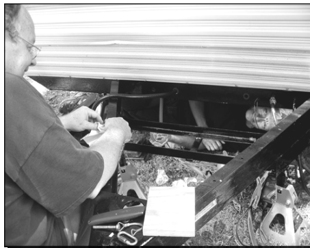
Lowell & Jim installing a heavy duty electrical system on the trailer.
