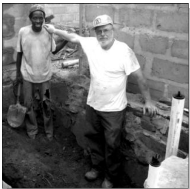
Terry spent much of his time "in the trenches" doing plumbing.
