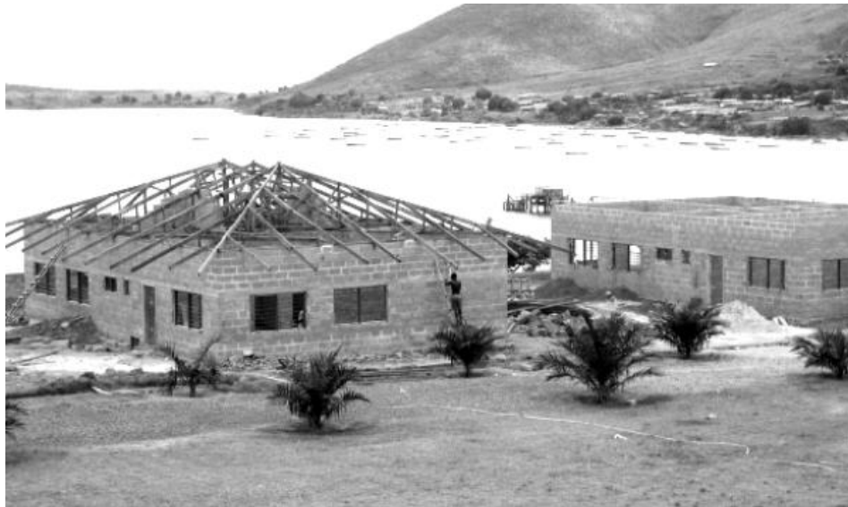
Construction has begun on two new guest houses.
