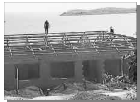
Ready for Metal Roofing
